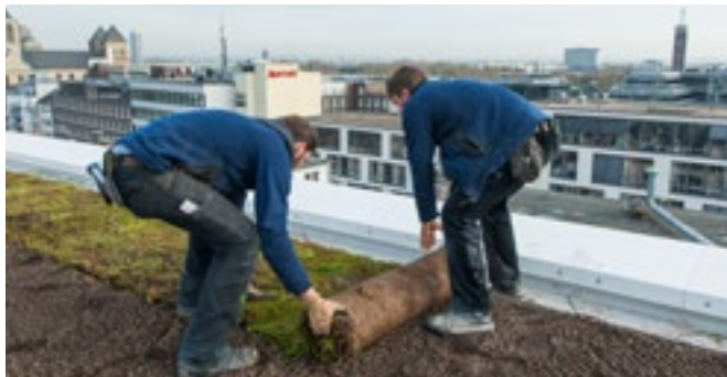
Installation of the vegetation
