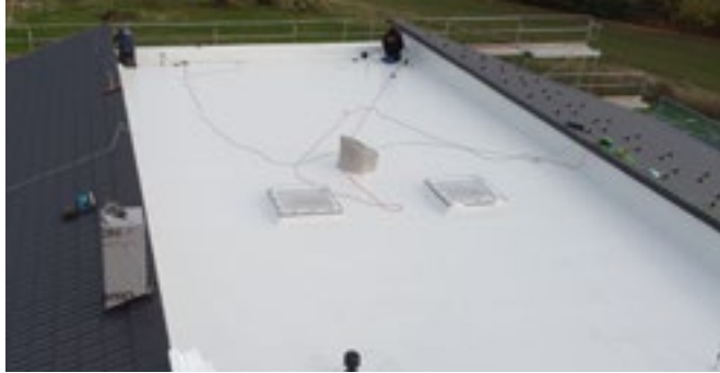
Installation of KÖSTER TPO waterproofing membranes
