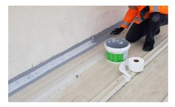
For inside and outside corners, first apply a coat of the KÖSTER MS-Flexfolie. It is recommended to secure the corners by adhering a circle patch using the KÖSTER Superfleece with approx. diameter of 8 cm as shown in the figure to the fresh coat of the KÖSTER MS-Flexfolie. Apply the second layer of KÖSTER MS-Flexfolie "fresh in fresh".
