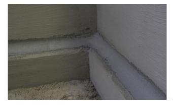
Install fillets (leg length of approx. 4 – 6 cm) made from KÖSTER Repair Mortar Plus at least 24 hours before applying the first coat of the KÖSTER MS-Flexfolie.
