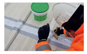
the reinforcement layer must be achieved. The fleece reinforcement must be completely covered with KÖSTER MS-Flexfolie and the KÖSTER MS-Flexfolie extended a minimum of 5 cm beyond the fleece. Make sure there is no air entrapped in the KÖSTER Superfleece.
